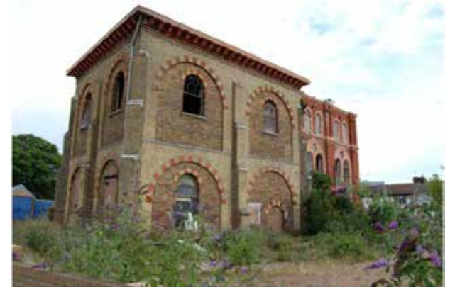
Rear view of the pumping station
