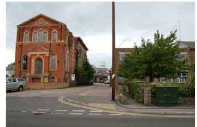
Unlisted pumping station and adjacent offices, fronting Trinity Road
