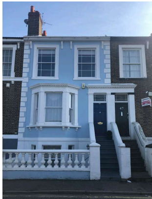
Decorative brackets under eaves
